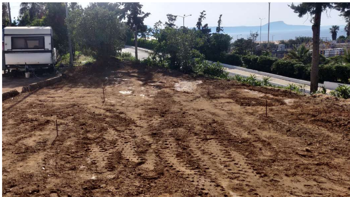
Preparatory works for the construction of the concrete base
